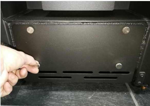
Picture 1: Remove the screws and the cover plate to locate the baffle plate.
